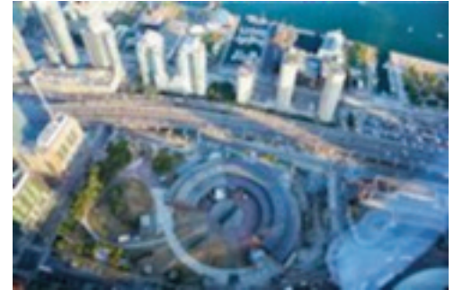
View from the CN Tower of the Locomotive Roundhouse
